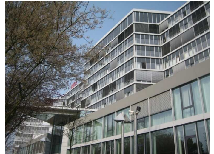
The renovated GTZ main building
