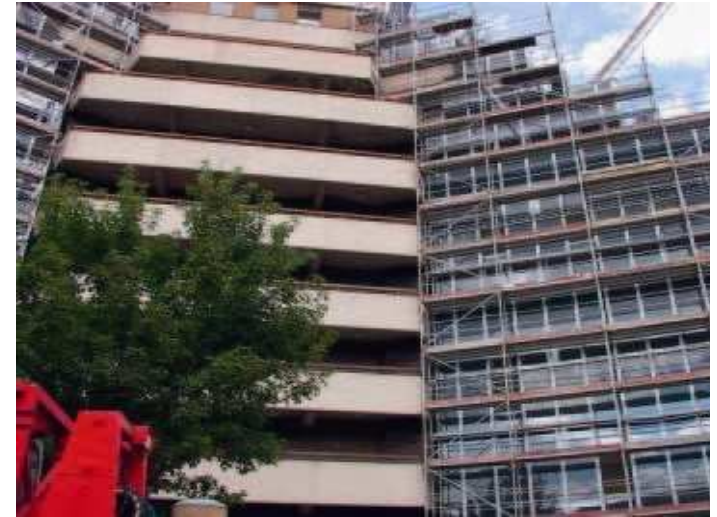
GTZ main building during renovation
