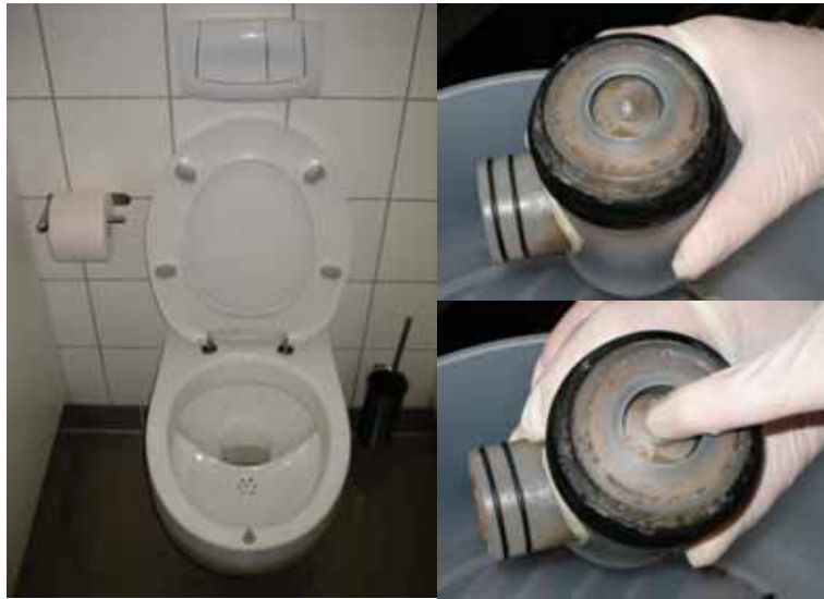
50 low-flush urine diversion toilets (Roediger) (1-3 L per urine flush, 6-9 L per faeces flush). Set during installation
