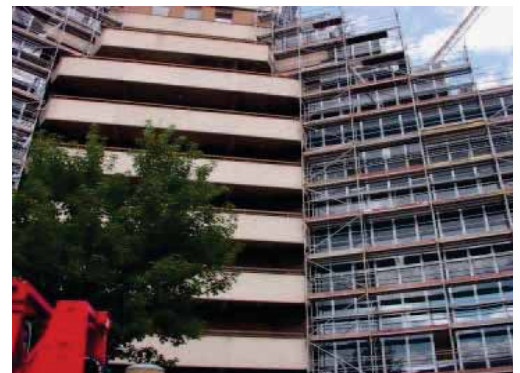
GTZ main office building during renovation
