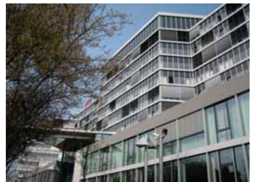
The renovated GTZ main building
