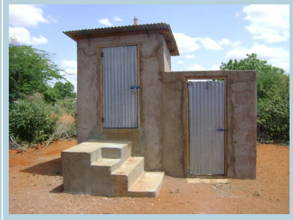
UDDT design in dry northern part of Kenya with attached shower
