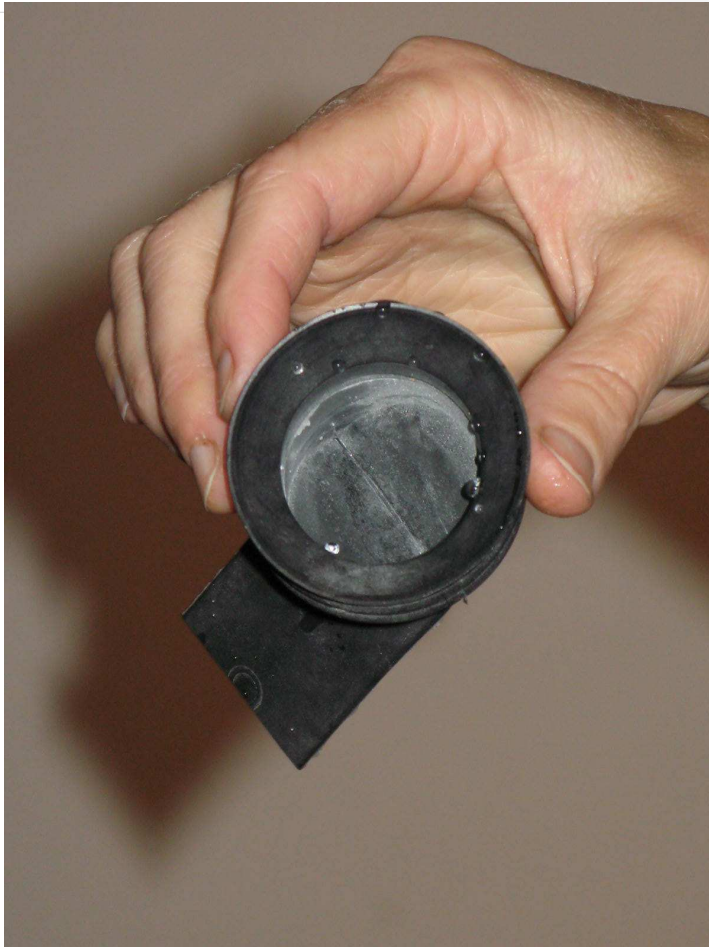
Flat rubber tube in Keramag waterless urinal
