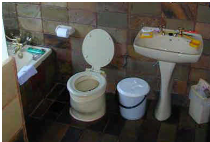
Figure 1: Dry ecological sanitation can be made comfortable and look urban, but there may be an emptying and collection problem and surviving germs.
