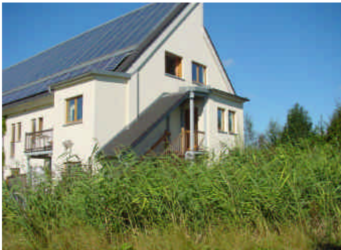
Figure 3: View on the subterra reed-bed and the solar equipped house
