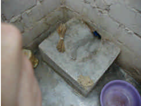
Figure 3: Luanda dry latrines are converted to pour flush, and they are impressively clean.
