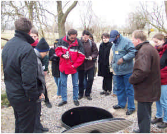
Manhole in sewerage system, excursion
