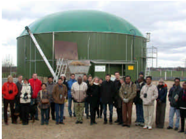
Farm scale biogas plant in Bornhöved, excursion
