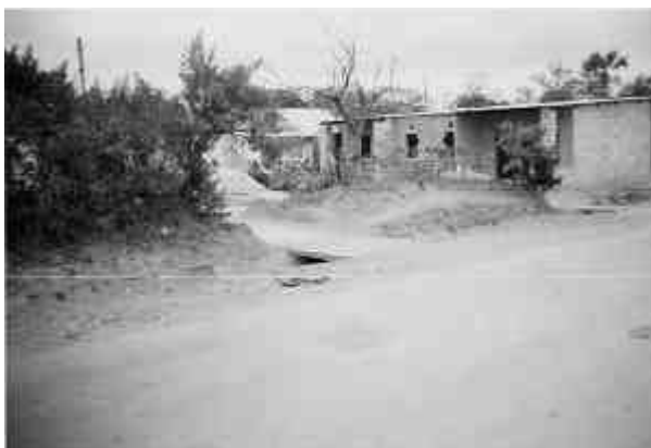
Figure 2: Building extensions, source: field data 2002
