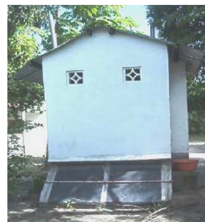
Figure 2: Public latrine with drying chambers (source: PAARSS)
