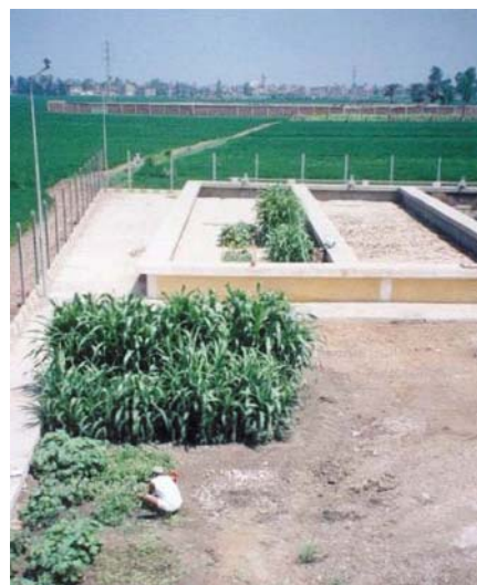
Figure 5: Conversion work in Navaq (source: ipp consult )
