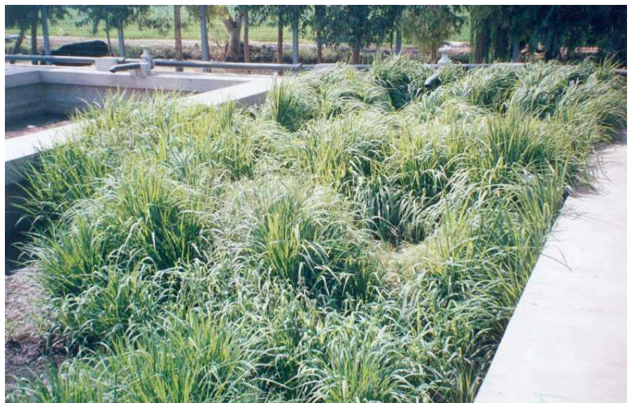
Figure 1: Sludge conversion polder planted with grass in Nawaq (source: ipp Consult)
