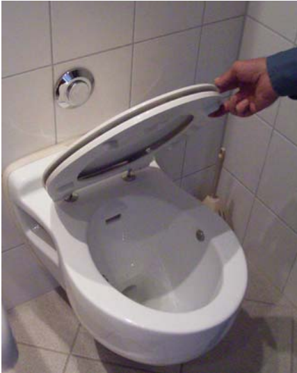
Figure 3: Vacuum toilet (source: Otterwasser)
