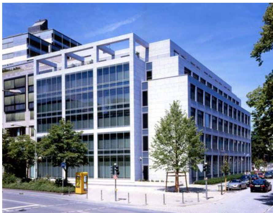
Figure 1: KfW building "Ostarkade" in Frankfurt am Main, Germany (Photo: KfW)
