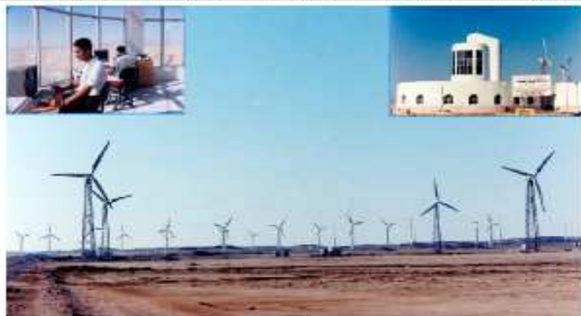
(Fig. 5) A side view of Hurghada wind farm and wind technology center
