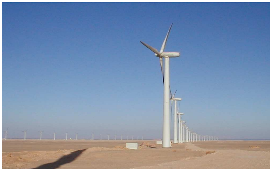
Foto taken during construction 1999/2000
