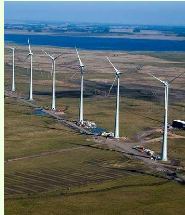
Osório Windfarm, Rio Grande do Sul State 75 x E-70/2000 kW = 150 MW, 98m concrete towers Owner: Ventos do Sul/Enferin/Elecnor Customer: Eletrobrás/CEEE (energy supply)
