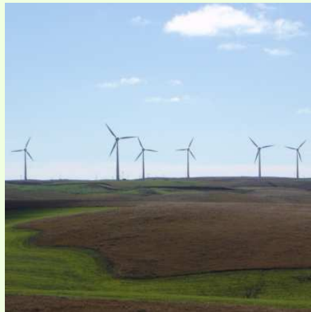
Horizonte Windfarm, Santa Catarina State 8 x E-40/600 kW = 4.8 MW Owner: CENAEEL Customer: CELESC (energy supply)
