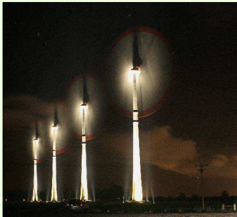
Osório Windfarm, Rio Grande do Sul State 75 x E-70/2000 kW = 150 MW, 98m concrete towers Owner: Ventos do Sul/Enerfin/Elecnor Customer: CEEE (energy supply)
