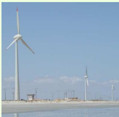
Macau Windfarm, Rio Grande do Norte State 3 x E-40/600 kW = 1.8 MW Owner: PETROBRAS Customer: Self-Generation
