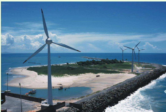
Mucuripe Windfarm, Ceará State 4 x E-40/600 kW = 2.4 MW Owner: WWP Customer: COELCE (energy supply)
