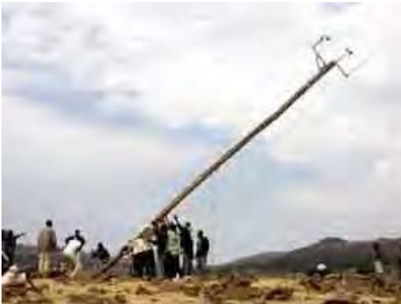
Figure 2-9: Bilagig, Gondar - Erecting the Pole
