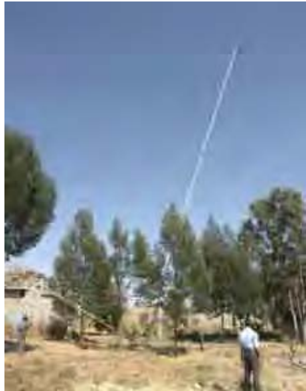
Figure 1-13: Dismantling of EREDPC 30 m Tower 19
