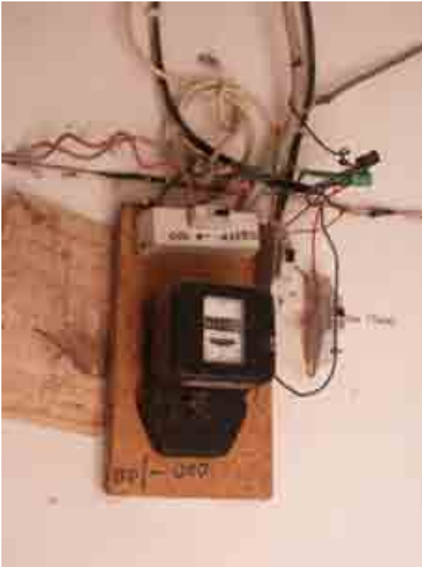
Figure 5-1: Typical House Connection with kWh-meter
