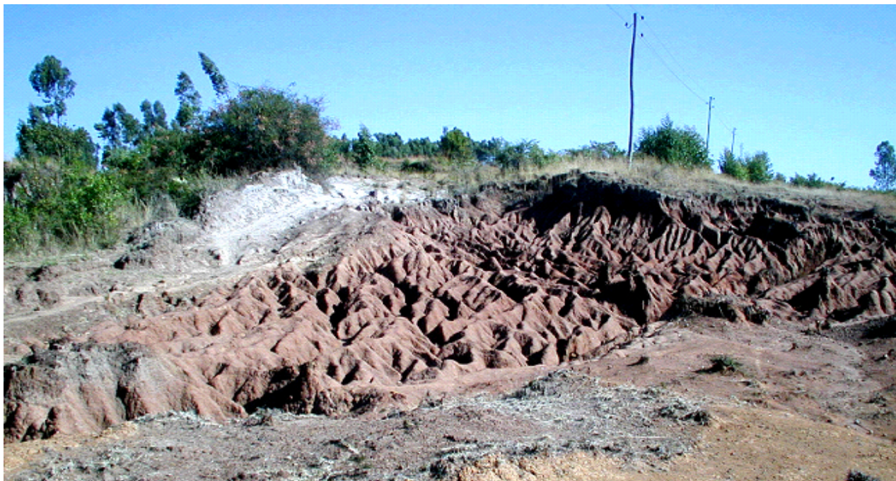
Figure 3-7: Soil Erosion close to Hydro Power Reservoir
