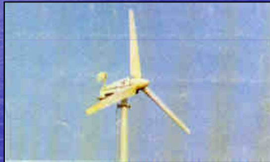
25 Kw wind turbine with wooden blades placed on tubular tower of 15m height
