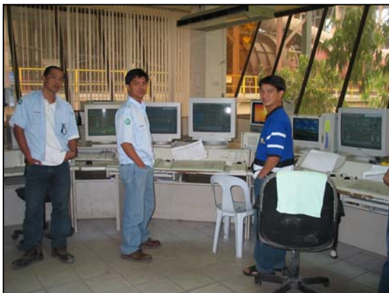
The control room of the cement plant
