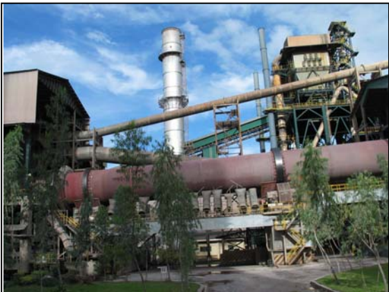
The Bulacan cement plant
