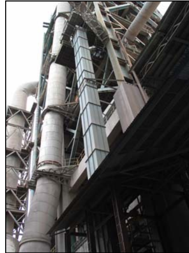
The conveyer runs in the angular tunnel
