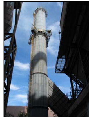
The chimney with the monitoring platform
