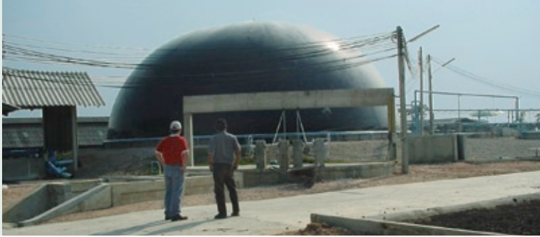
Before the biogas programme started, the agro-related businesses had been discharging waste and waste water into ponds.
