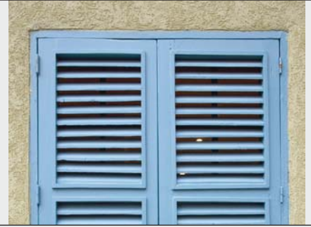
Addis Ababa, Kasanches Palazzine Windows after renovation
