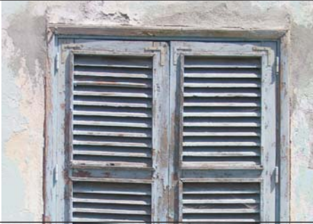
Addis Ababa, Kasanches Palazzine Windows after renovation
