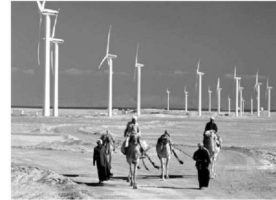
Zafarana wind farm, Egypt
